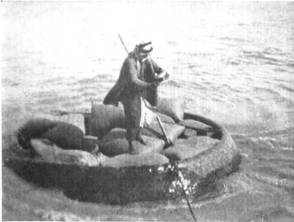
FIG. 135. A GUFU OR REED BOAT PITCHED WITH BITUMEN.
