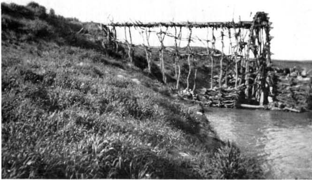
FIG. 66. MESOPOTAMIAN WATER-WHEEL.
